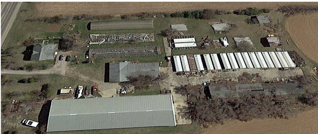
Photograph 8: Aerial photo of 1052 Colborne Street West (Source: Google Earth)
