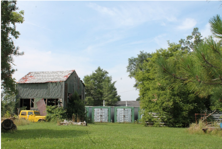
Photograph 9: Barn and kilns at 1052 Colborne Street West
